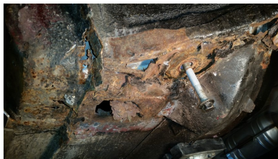
Cleaned up, the extent of the rot was visible
