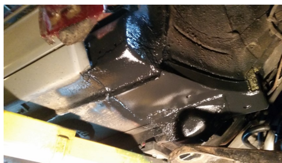
Welded up and looking good
